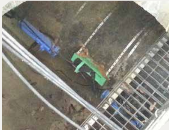
Foreign Ultrasonic Transducer (Green) and Jain Technology Ultrasonic Transducer(Blue) (K-Water Profit Sharing Task 2014)
