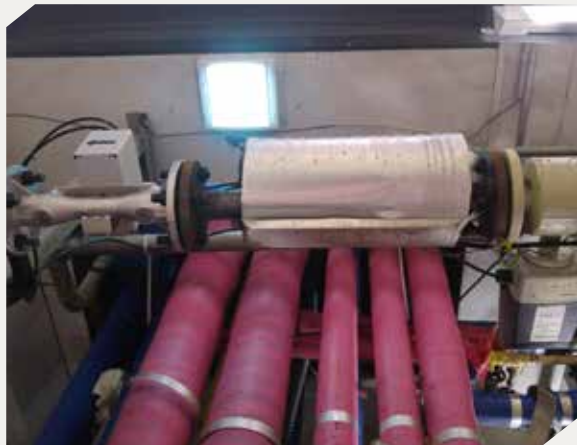
Korea District Heating Corporation (Xonic 10LE)
